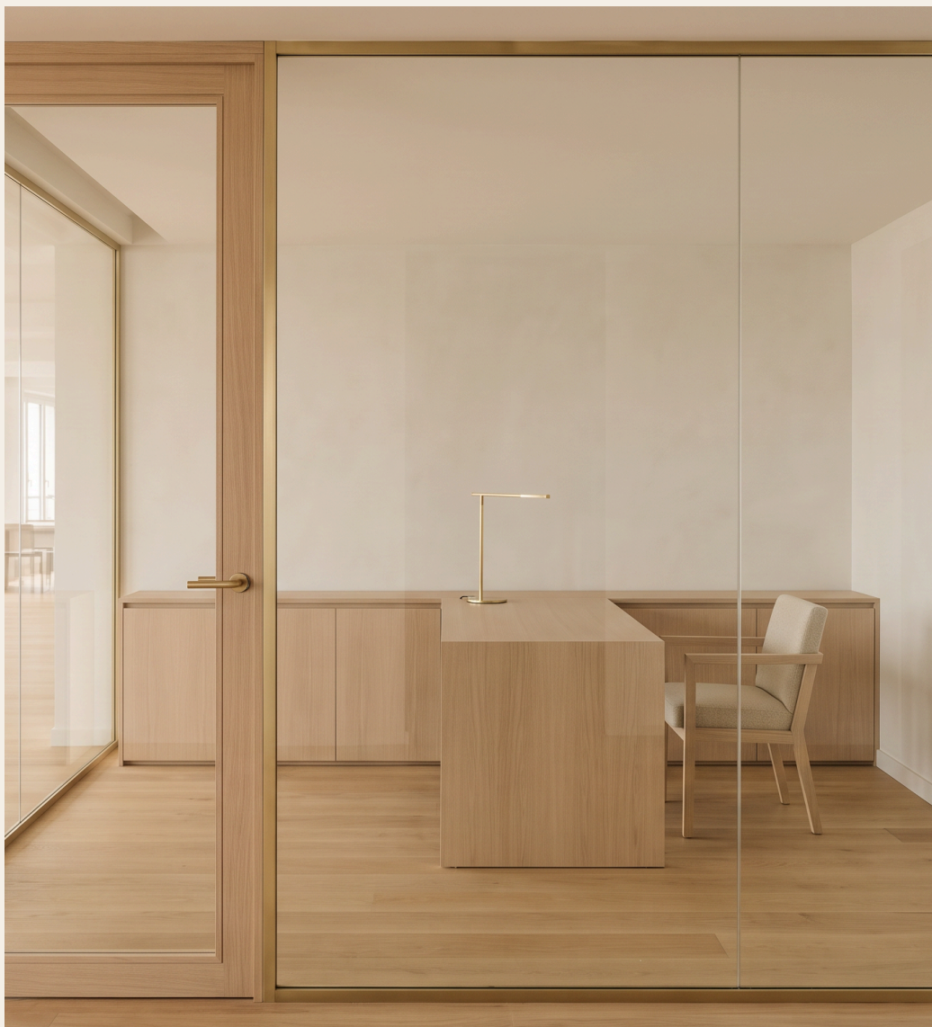
PART-GLAZED PARTITION · BORROWED DAYLIGHT
