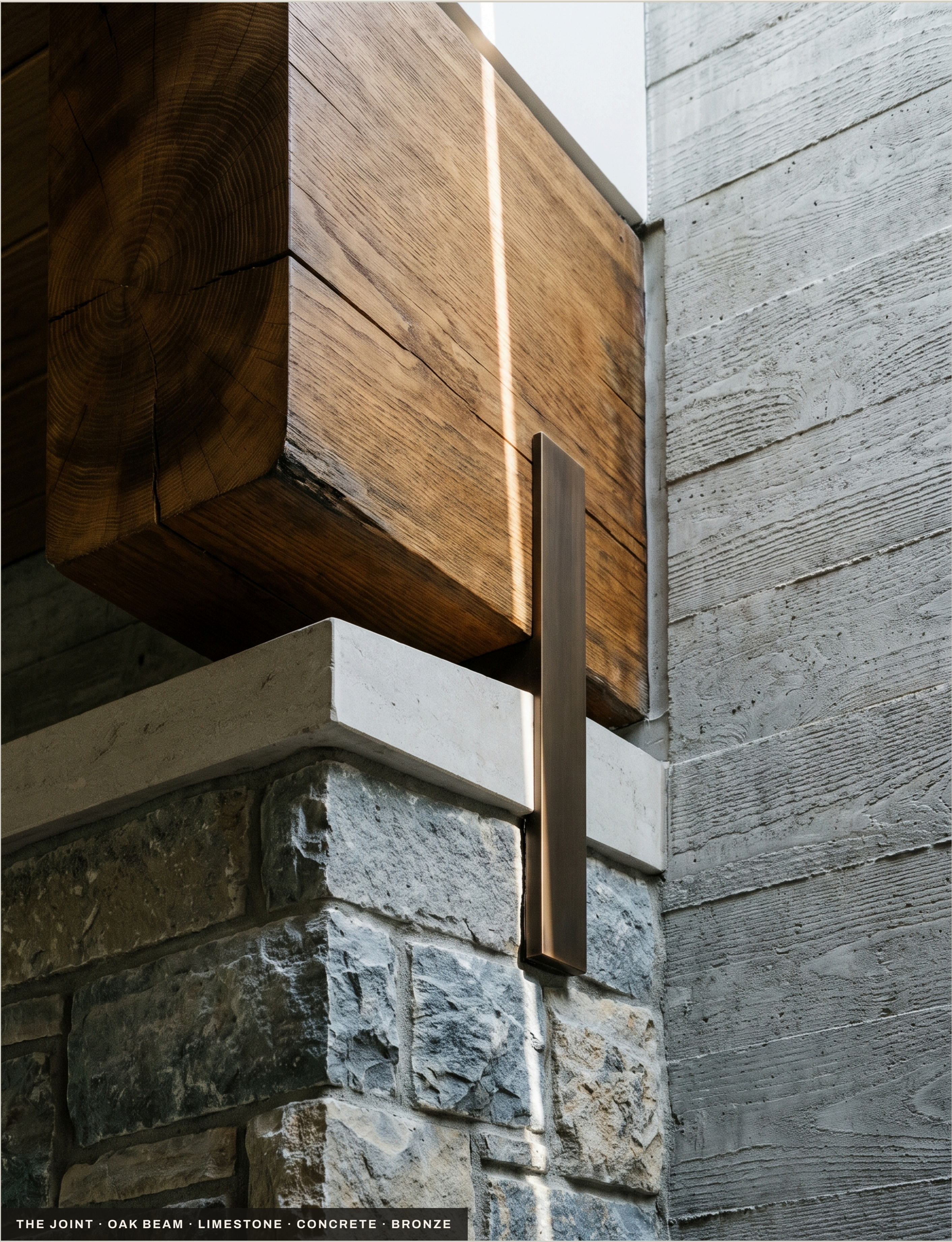
THE JOINT · OAK BEAM · LIMESTONE · CONCRETE · BRONZE
