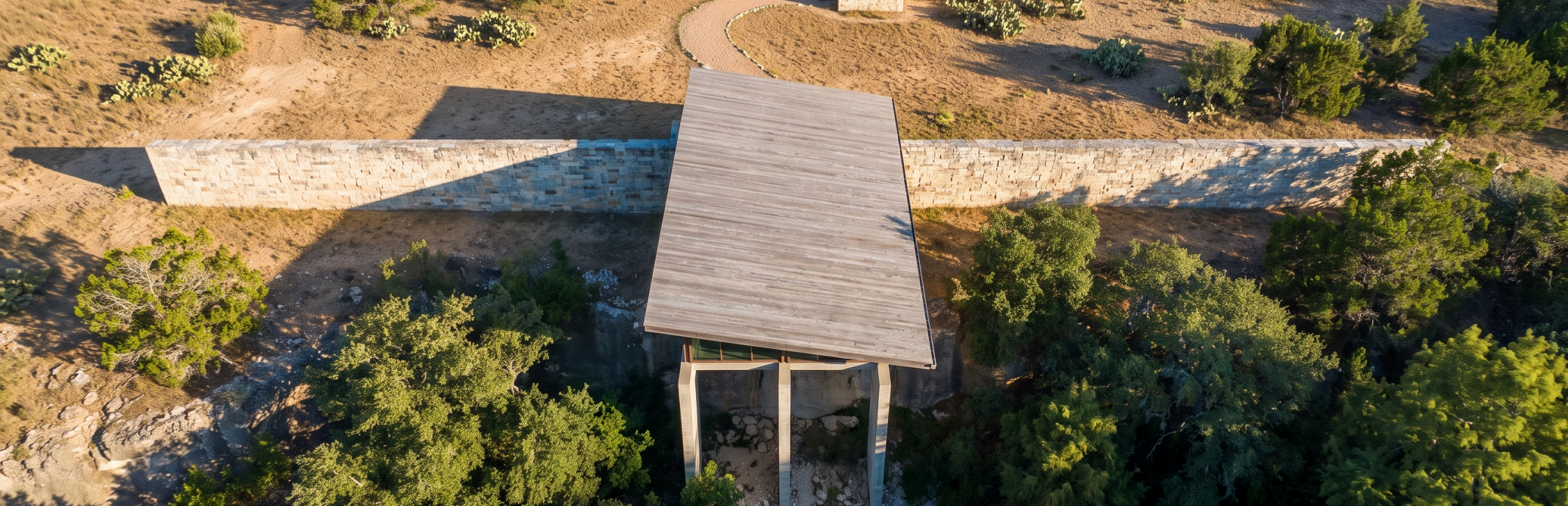
FIG. 01 — THE SITE FROM THE NORTH-WEST. The wall lies east–west along the caprock edge; the hall reaches north off it and cantilevers over the green ravine on a single row of piers. Plateau in warm sun, ravine in green shade — the site's two conditions in one frame.
